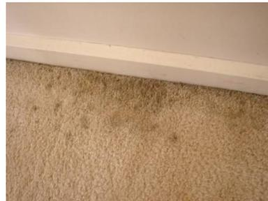
Tell tale signs of a broken pipe/leaking water to a wall adjacent or inside/behind the wall.
